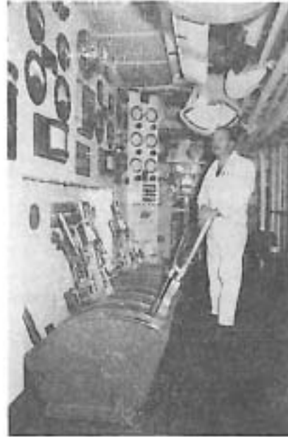
Ship's engineer at controls in engine room of Princess Marguerite.
