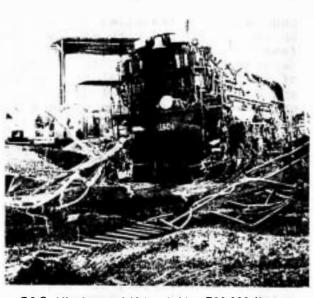
C&O Alleghany #1604 weighing 750,000 lbs. was washed against the concrete bridge pier causing extensive damage to the cab area. If the bridge pier had not stopped it the locomotive would have toppled on it's side,
