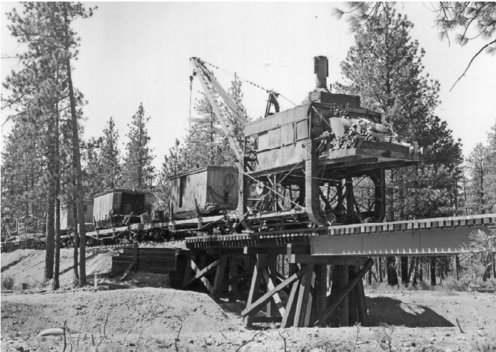
Above: A Brooks-Scanlon Lumber Company loco eases a string of log cars across a trestle in the pine country near Bend, Oregon. Left: It was moving day on Brooks-Scanlon when the photographer captured this view of a train with several skid shacks on log cars and a swing-boom McGiffert loader being pulled to a new location. *Photos, Jack Holst collection, PNWC-NRHS Archives*
