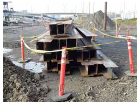
Below right: Steel piles will be used for the site because it was determined that the ground was too porous to use cast-in-place concrete piles. (January 13 photo by Arlen Sheldrake)
