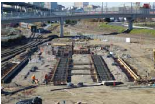
Below: Notice the amount of re-bar necessary under the engine tracks. The string of passenger cars at the left includes the Chapter's Mt. Hood. (March 8 photo by Arlen Sheldrake)
