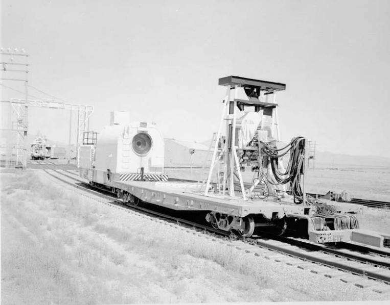
Snaptran-2 experiment mounted on dolly being hauled by shielded locomotive from IET towards A&M turntable. Note leads from experiment gathered at coupling bar in lower right of view. August 25, 1965, INEEL Negative no. 65-4503; used with permission from INL; photo from Library of Congress HAER ID 33-E-49
