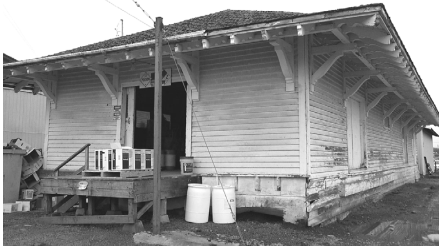
North end of Depot, Benton County 2006 photo provided by Chris Bentley
